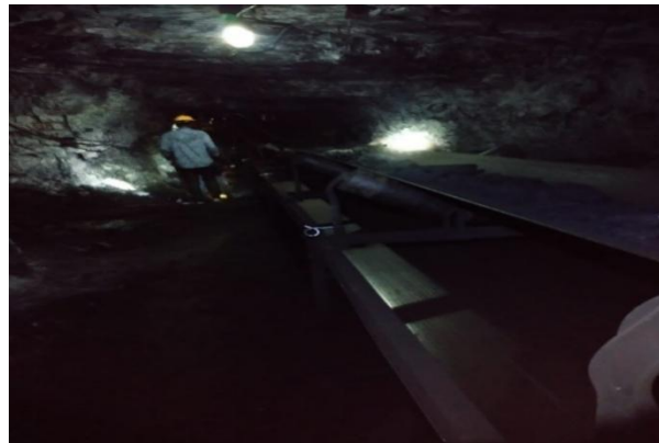
Figure 5.5 Belt conveyor system handling coal
