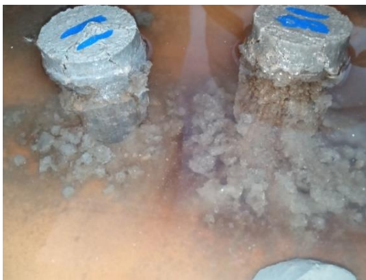
a) Soaking of specimens in water
