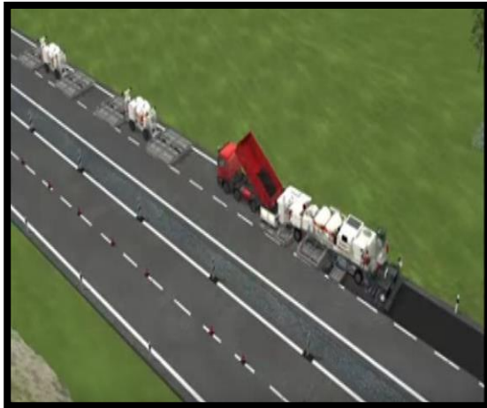
a. Preheater and Milling Units
