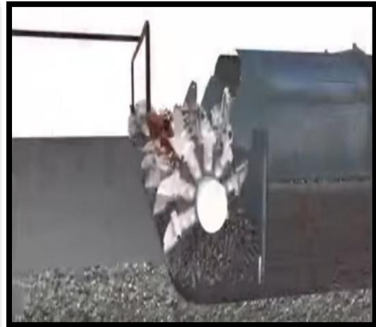
b. Milling of the top surface of the pavement
