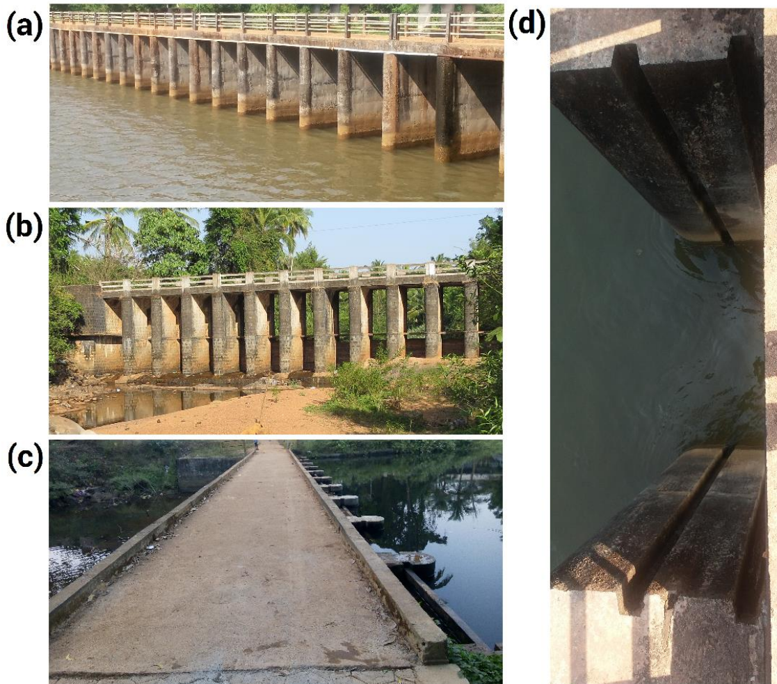
Figure 1.3 A view of Vented Dams across the Pavanje River; (a) Downstream of a unregulated Vented Dam (b) Downstream of a regulated Vented Dam (c) View of both upstream and downstream of a regulated Vented Dam (d) Pair of grooves incised within the piers to stack the timber panels for flow regulation
