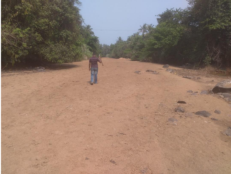
View of Streambed between Vented dam 1 and 2
