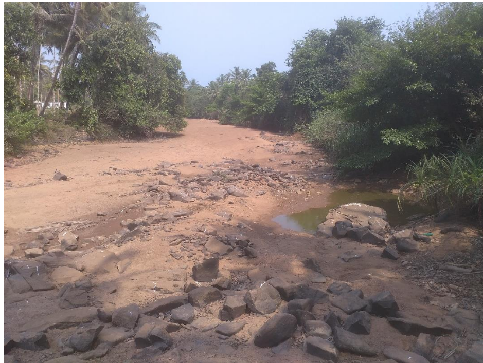
View of Streambed upstream of Vented dam 2
