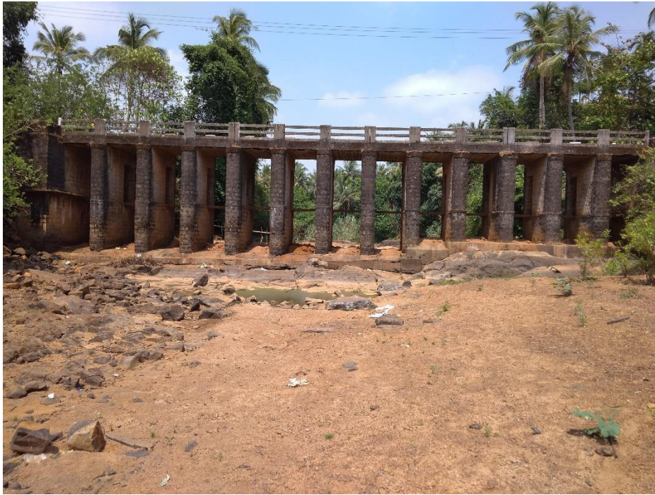
View of Vented Dam when gates are open in the month of May 2016
