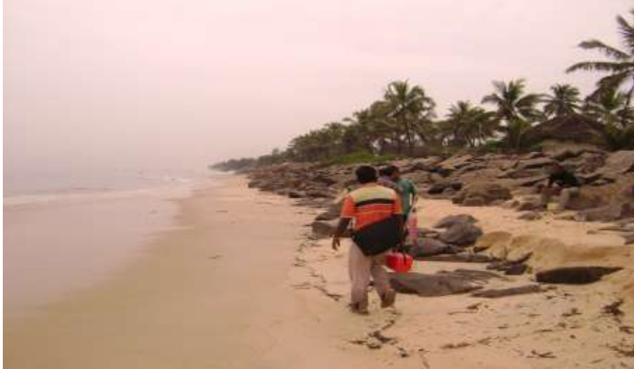
Plate.1 Protection by Sewall at Mukka Beach
