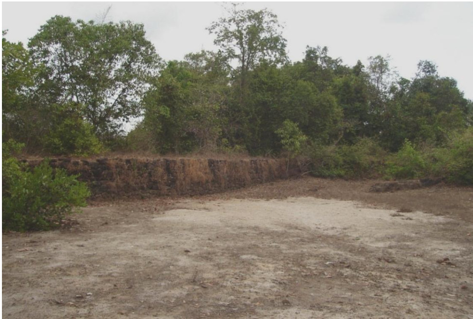
Fig. 9.1 Photograph of the silted tank under investigation at Nitte village
