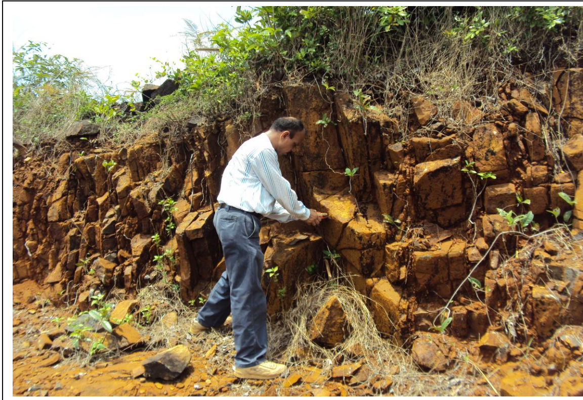
Fig. 3.26 Photograph showing the different sets of joints in the gabbroic mass
