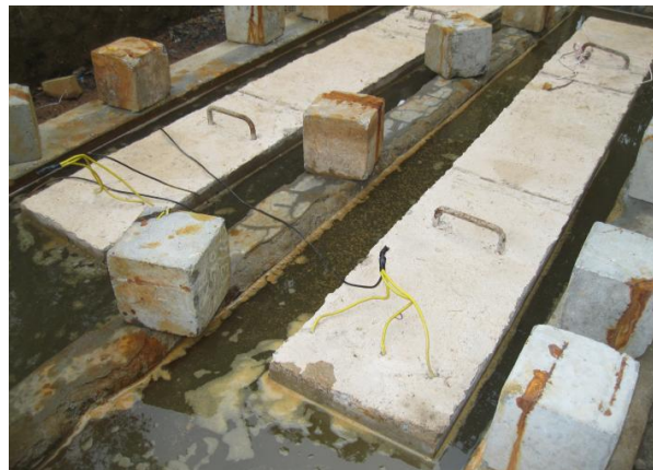
Fig. 3.5(b) Accelerated corrosion of beam specimens
