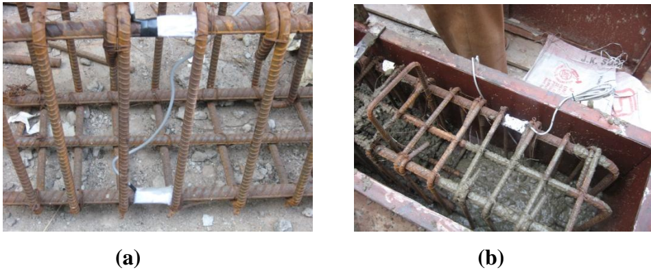
Fig.3.13 Fixing of strain gauges on the rebar
