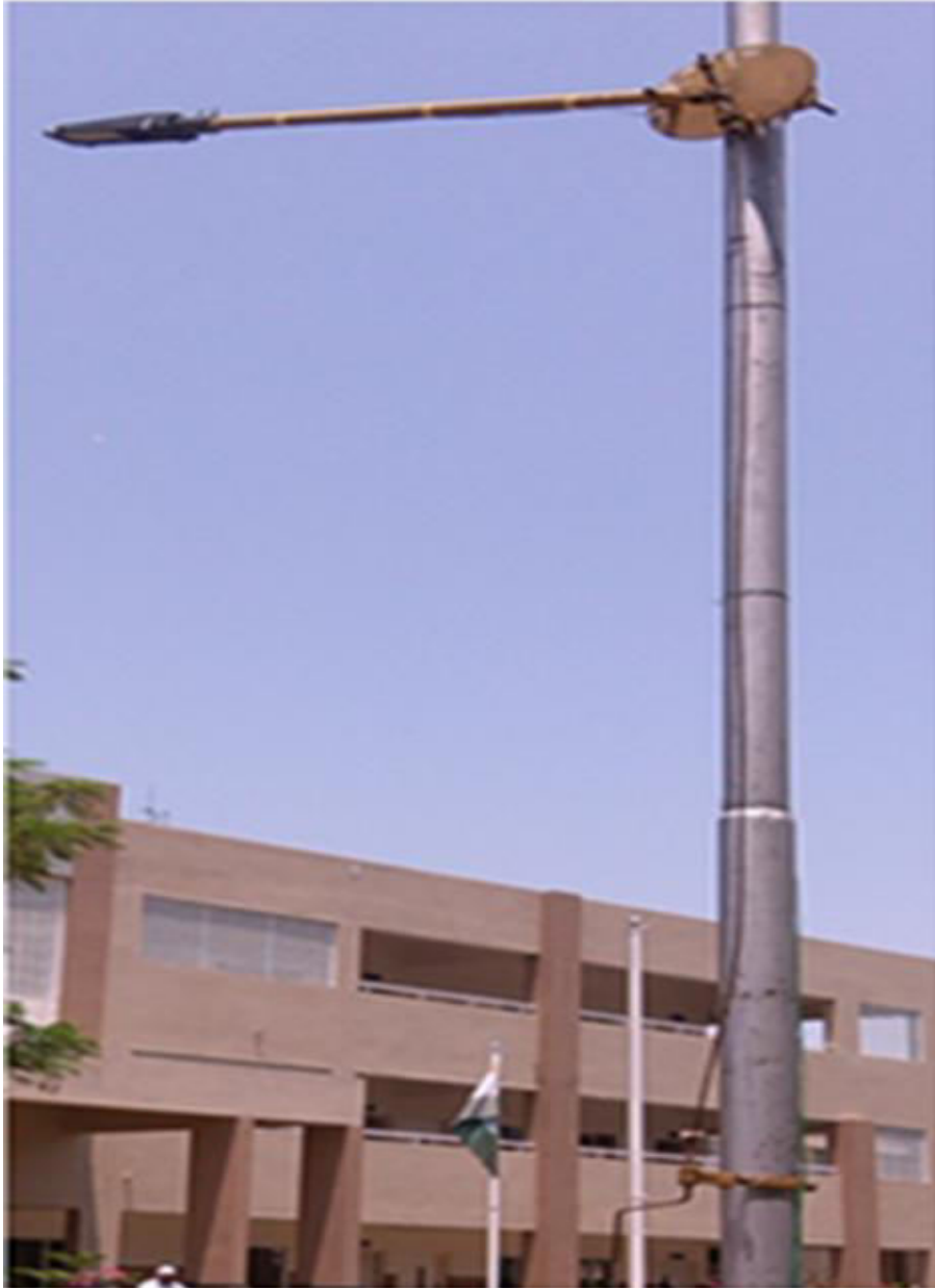
Fig. 4.4 Fabricated light pole
