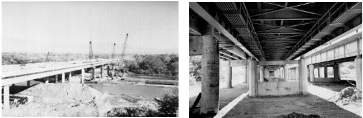
Fig. 4.22 General view of I – 40 Bridge
