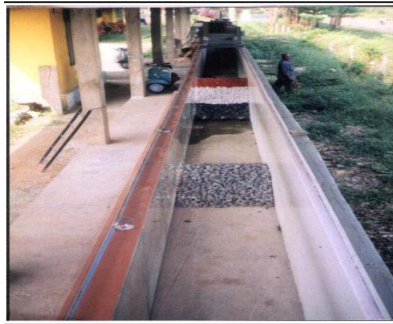
Plate 3.6 View of protected breakwater
