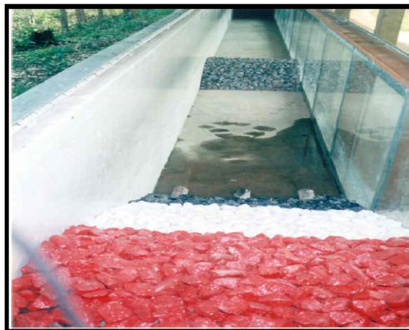
Plate 3.7 Top view of protected breakwater
