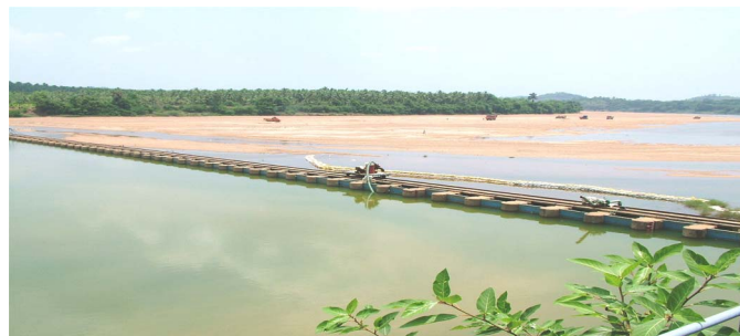
Fig. 2. Existing vented dam at Thumbe across the Netravathi River
